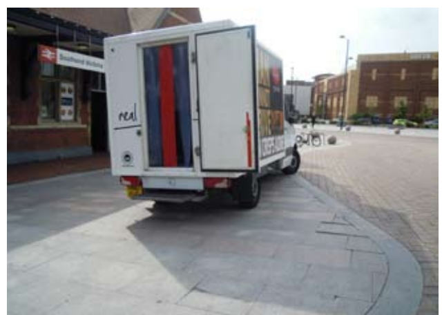
Delivery vehicle outside station western entrance - large vehicles in inappropriate locations have damaged slabs
