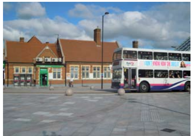
View north across vehicle path towards southern station entrance
