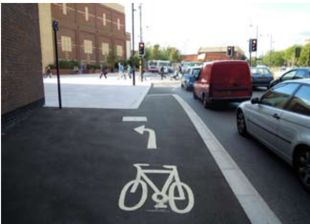
End of westbound off-carriageway cycle track and feeder into shared pedestrian/cycle southern hard-paved space
